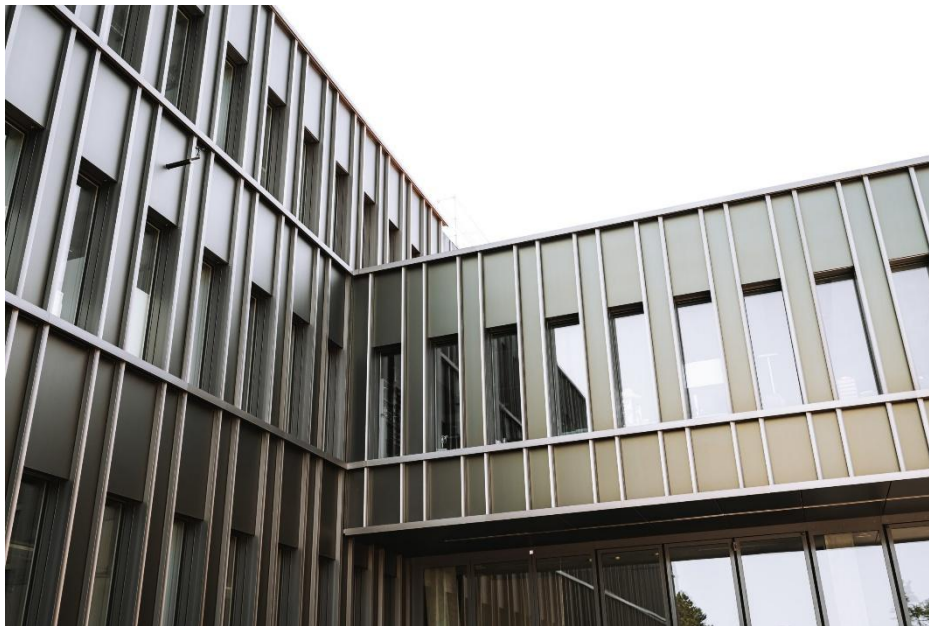
Figure 3.2-5 Example of angular colour stability of Kromatix panels.
