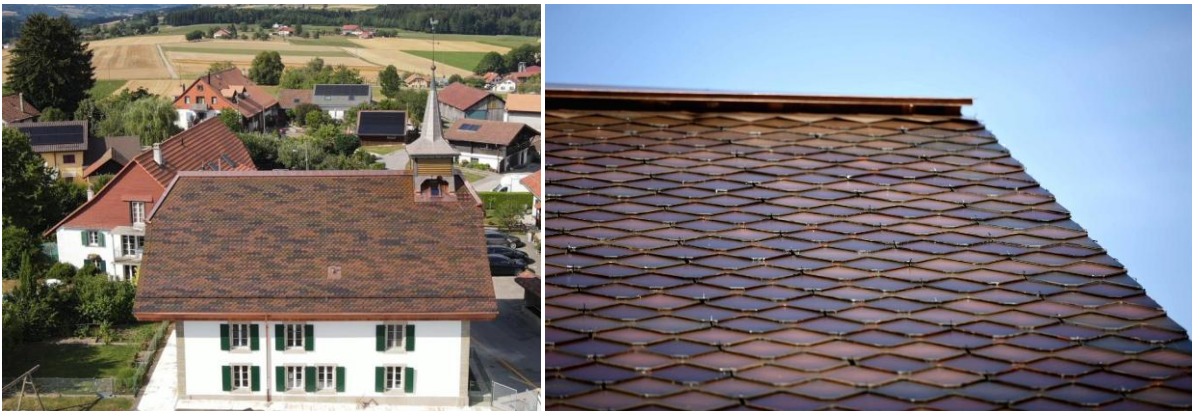
Figure 3.2-3 Freesuns project in Ferlens, Switzerland, with different tones of terracotta solar tiles.
