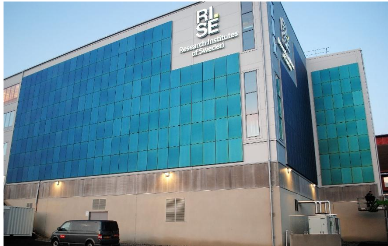
Figure 3.2-6 Example of colour reproducibility of Kromatix™ Blue Green. Small colour differences can be observed. It does give the façade a more natural look.
