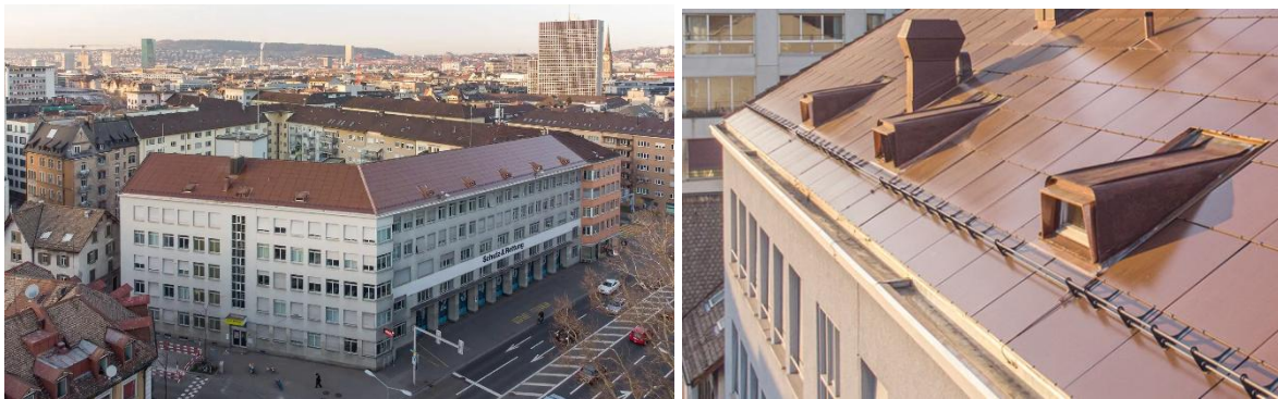
Figure 3.2-4 BIPV building in Zürich made with a Solaxess [32] film and implemented by 3S Swiss Solar Solutions AG [89].
