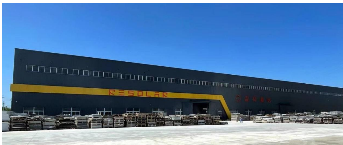
Fig. 2.2-10 Anhui Fengyang 10 000-tonnes PV module recycling plant
