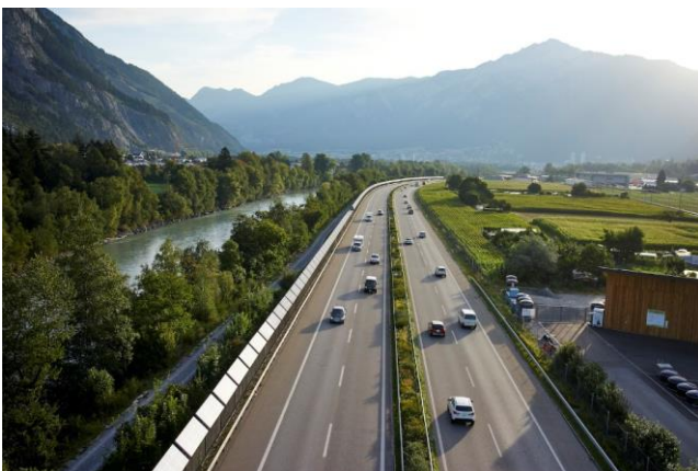
Fig. 11.1-2 PV sound barrier installation 100 kWp A13 (1989) 53
