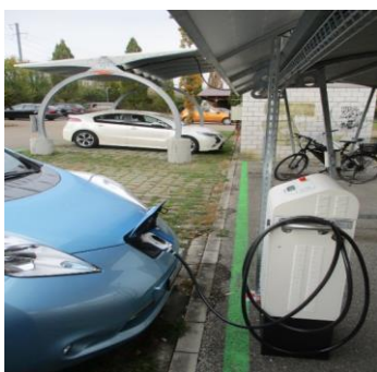
Fig. 11.4-1 Bi-directional EV at the PV Laboratory of Bern University of Applied Sciences BFH in Burgdorf, Switzerland 54 (Source: Muntwyler)
