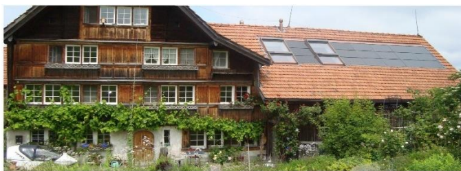
Fig. 6.6-2 Innovator with "in-roof grid-connected" PV installation, integrated hot water solar thermal installation and a TWIKE (left) in Switzerland before 2010 (Source: Solarcenter Muntwyler AG)
